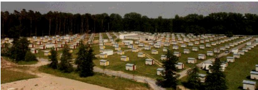
Fig. 3. KASCADE detector array with a field array, a central detector for measuring the hadron component and the muon component at various energy thresholds. In addition there is a muon tracking detector arrangement in a tunnel.
