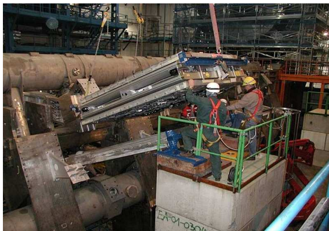
Fig. 7. Installation of a muon station (integrated MDT and RPC) into the Barrel Toroid.
