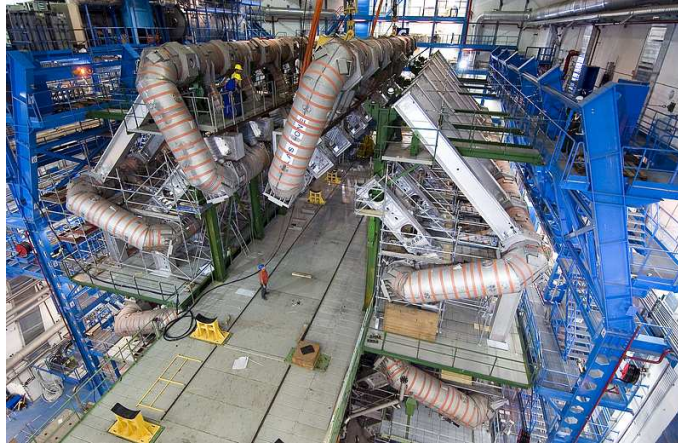
Fig. 2. Picture taken of the Barrel Toroid underground installation when the last coil was put into place on 25th August 2005.
